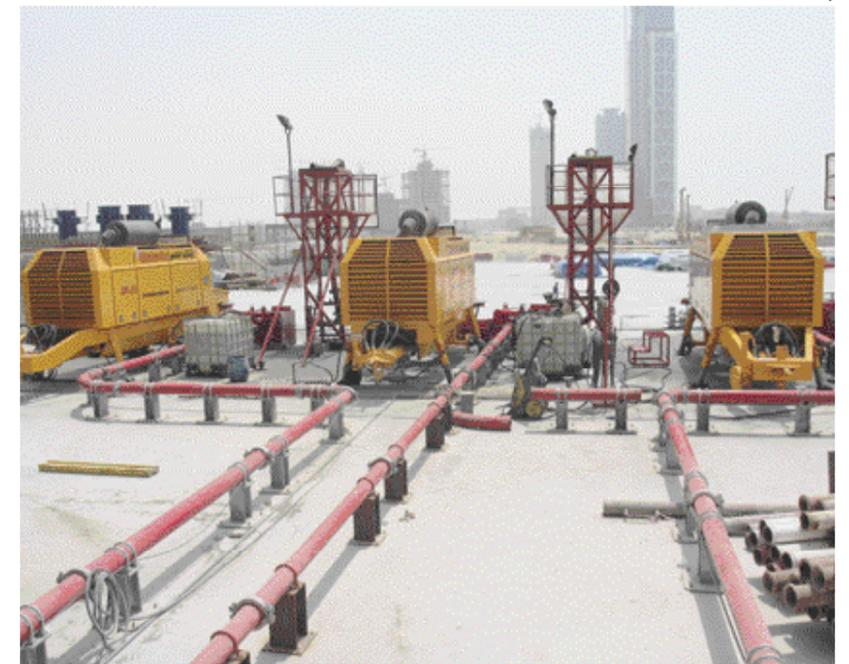
Overview of the layout of the delivery lines at the pump station – the two super high pressure BSA 14000 SHP D pumps are shown on the left and right
