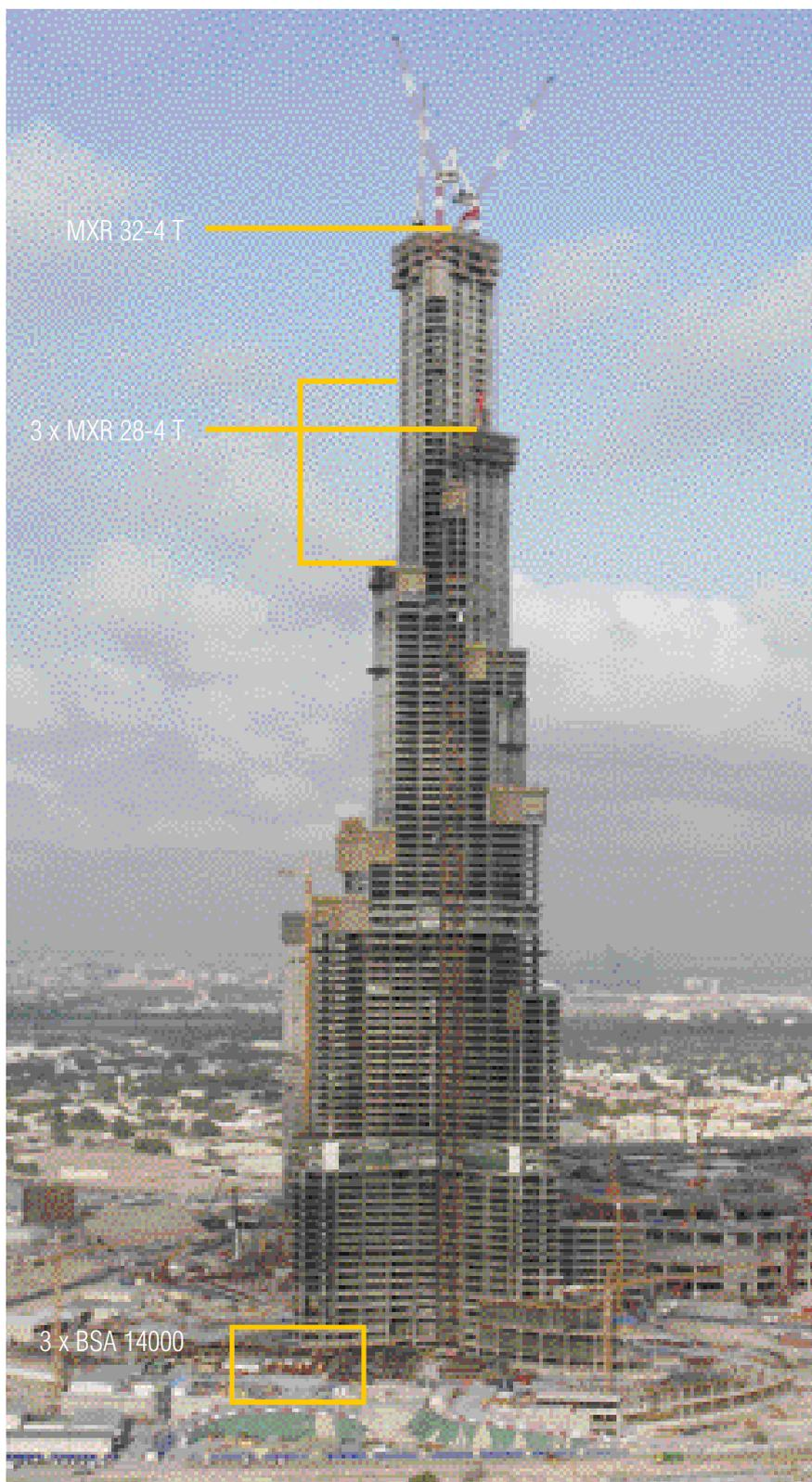
With several Putzmeister high performance concrete pumps, a sophisticated delivery line system, non-ballasted stationary booms and demanding concrete mixtures, the carcass of the Burj Dubai is currently under construction. The constructor, Emaar Properties (UAE), has commissioned a consortium managed by Samsung (Korea) together with BeSix (Belgium) and Arabtec (UAE) with carrying out the construction works on the prestigious high-rise project.
