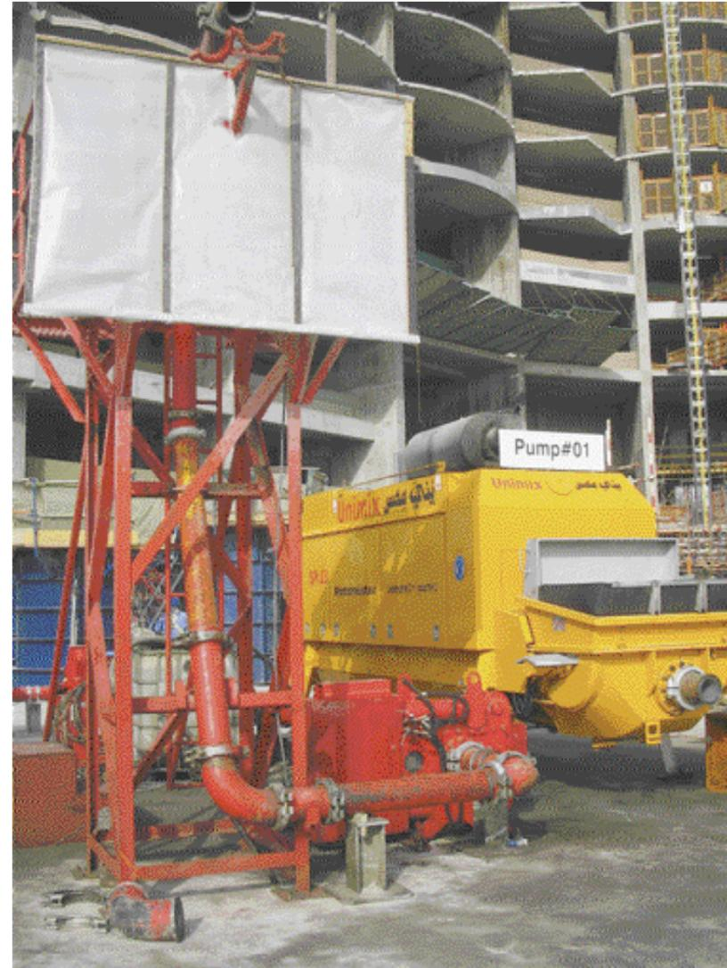
Structure of the cleaning station: on the right, one of the Putzmeister super high pressure concrete pumps, in the centre a shut-off valve with 90° pipe bend, which is either connected to the discharge connection of the concrete pumps for pumping operations, or to the connection for the cleaning tower
