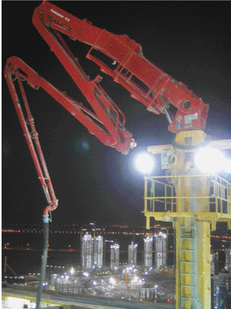
The non-ballasted Putzmeister MX booms do not pose an obstacle to backward walls nor other cranes on the formwork
