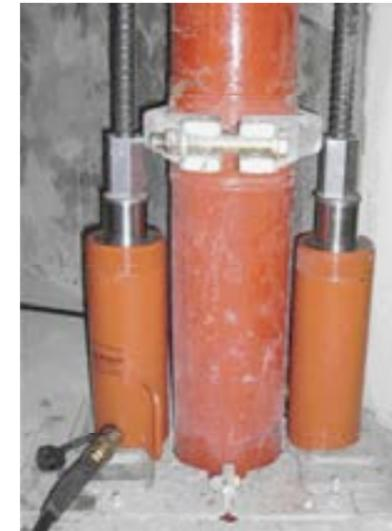
If individual pipes have to be replaced, the entire riser can be lifted by hydraulic cylinders
